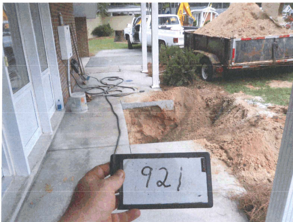
Picture 2: UST 921Barracuda excavation.
